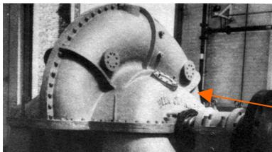
The DrKnock could be fitted almost anywhere on the pump housing since the noise resulting from cavitation travels through metal well.
